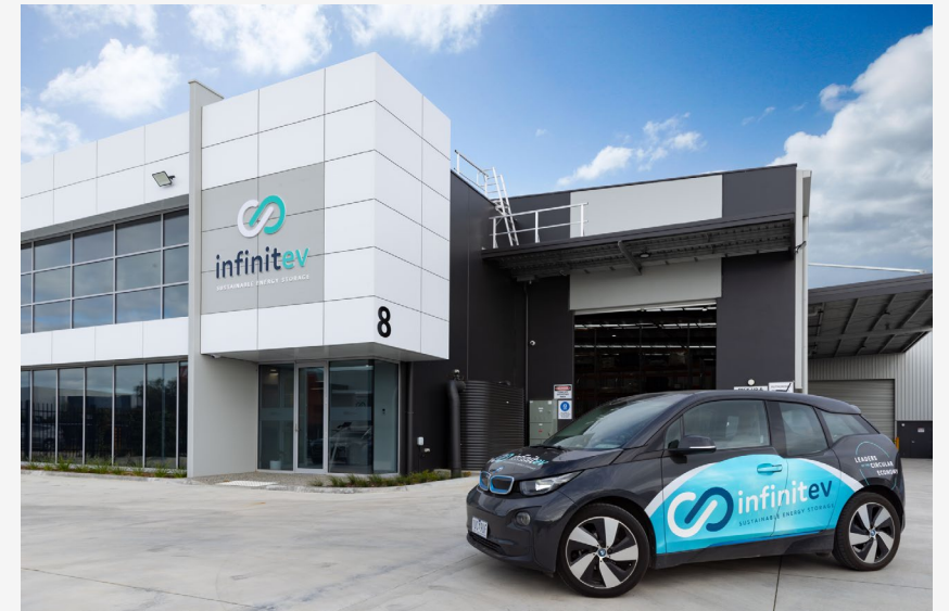
Infinitiv HQ and innovation centre located in Cranbourne, Victoria.
